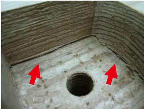
**Fig. 5. Wood depression and split at the bottom of the washer notches on the column member.**
